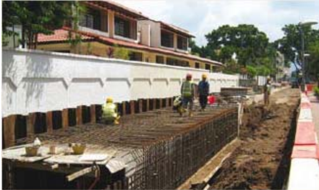
Improvement to Roadside Drains
