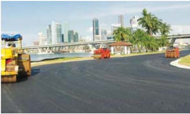
Road Works in City Centre Phase 2
