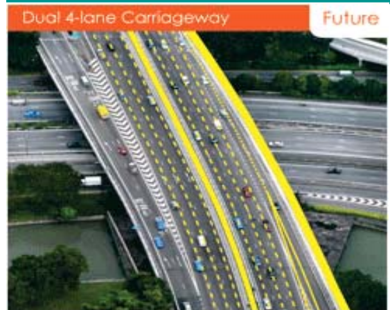
Fig6: Widened CTE Vehicular Bridge
