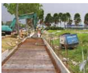
Final Premix Surfacing, Reinstatement and Ancillary Works at Tuas View, Phase 7
