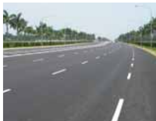
Final Premix Surfacing, Reinstatement and Ancillary Works at Tuas View, Phase 5
