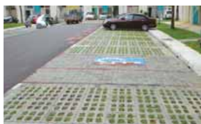
Carpark Improvement Works at Tampines Carpark No T37(Part), T41 and T42
