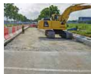
Final Premix Surfacing, Reinstatement and Ancillary Works at Tuas View, Phase 6
