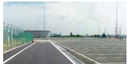
Civil Works 2 – New Polymer Storage
