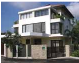
Proposed Erection of 9 Pairs of 3 Storey Semi-Detached Dwelling Houses at Woodlands Road
