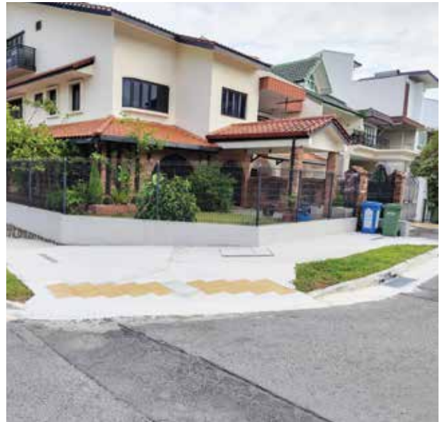
An ongoing OKP's maintenance project is the improvements to roadside drains at Eng Kong Place.
