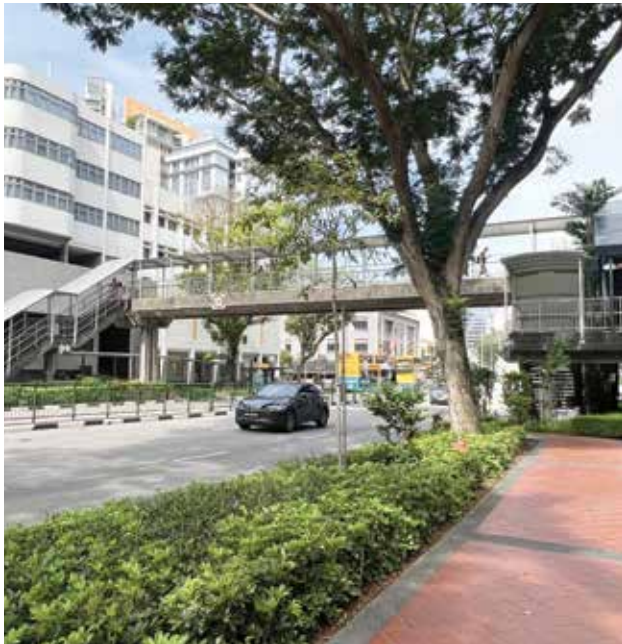
Covered linkway at Balestier Road is part of OKP's Commuter Infrastructure Enhancement project.
