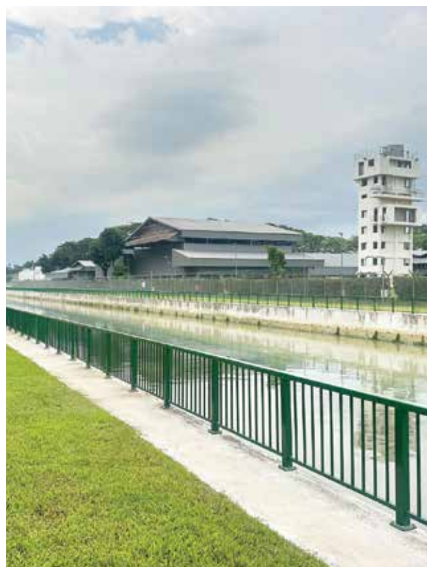
Another completed OKP's project was the improvement to Sungei Selarang.
