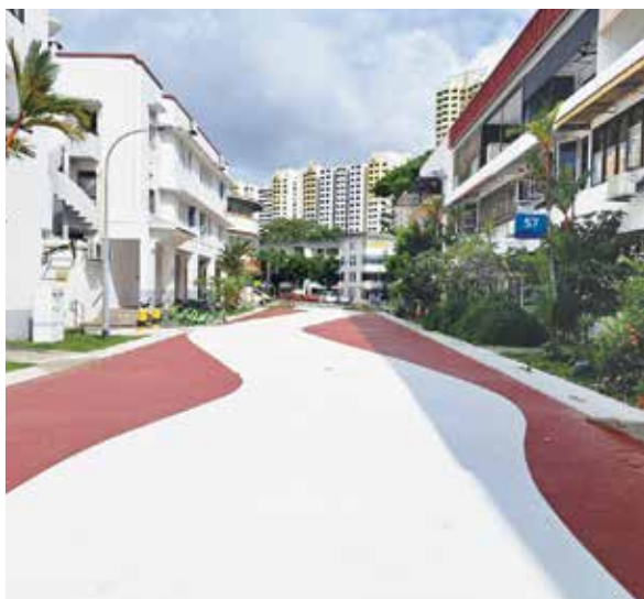
OKP completed road-related facilities and road repurposing at Eng Hoon Street.
