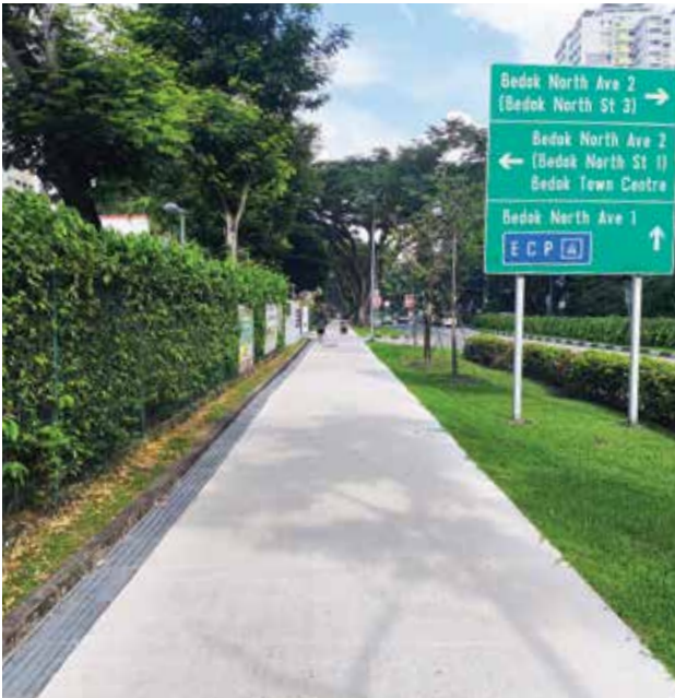
Footpath renewal is one of OKP's maintenance projects.
