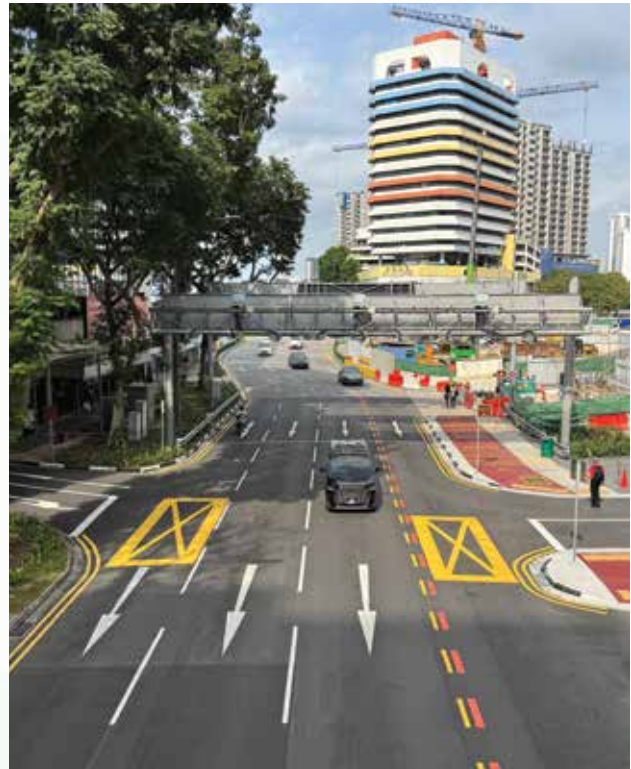
OKP is involved in the construction of Cycling Network (Central).
