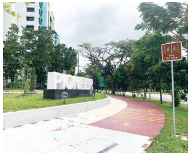
Construction of Cycling Path Network (West) at Upper Jurong Road is an ongoing OKP's project.
