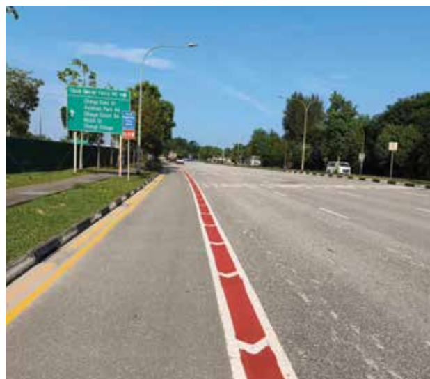
OKP completed the road maintenance contract for the South East Sector.
