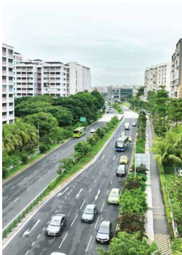
OKP completed the project involving commuter and road infrastructure works in Pasir Ris and Loyang.
