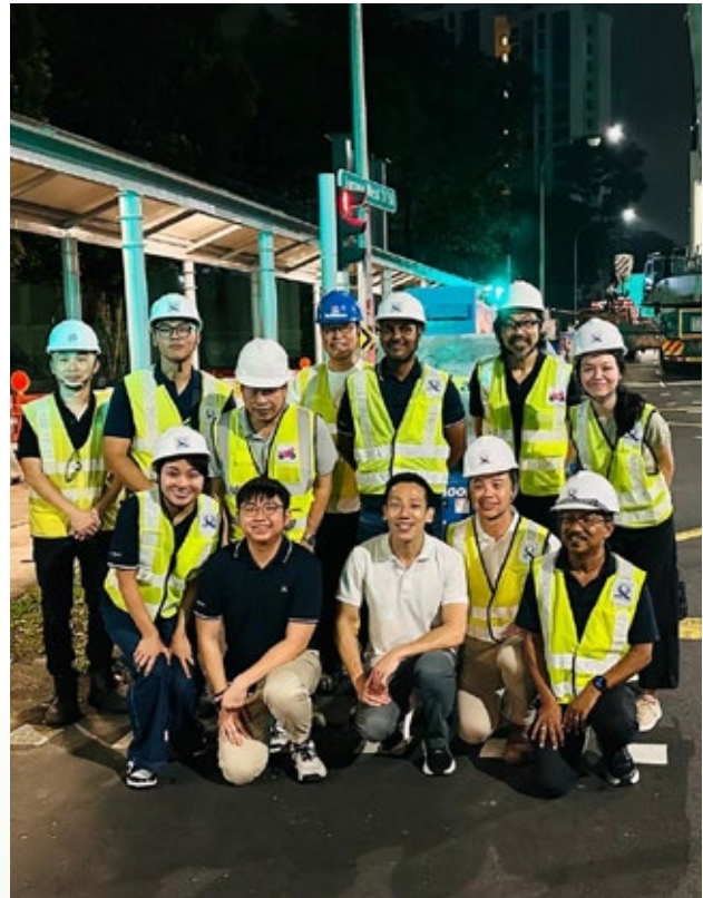
Successful Installation of the covered linkway across Jurong West Street 51, during an early morning visit by Mr Xie Yao Quan, Member of Parliament representing Jurong Central Single Member Constituency (third from right) on 21 June 2025.
