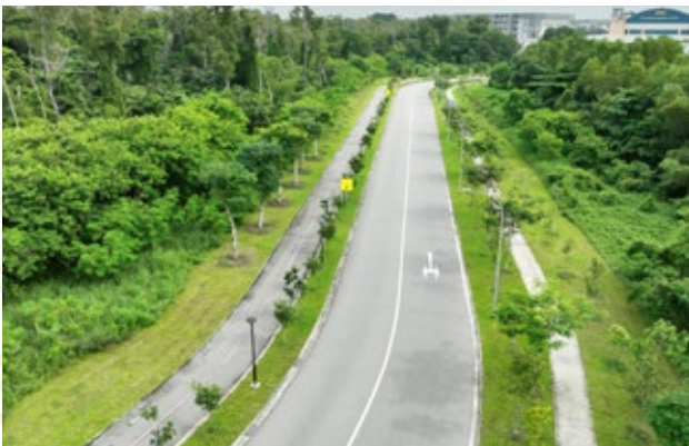
OKP completed its project involving commuter and road infrastructure works along a new road at Loyang Lane.
