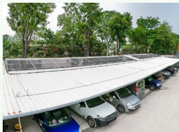
Solar panels at Jalan Papan site office.
