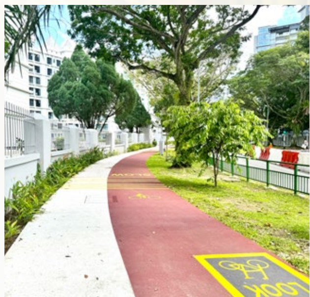
Completed cycling path using CMC at Serangoon Avenue 3.
