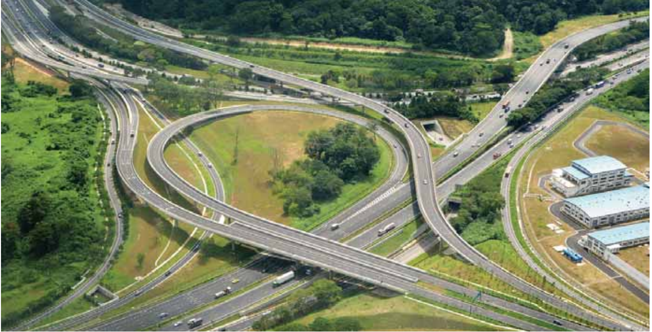
The expansion of the CTE/TPE/SLE Interchange is one of OKP's completed projects.
