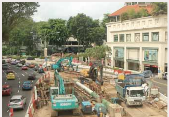
OKP is constructing the Stamford diversion canal – Tanglin and Kim Seng.
