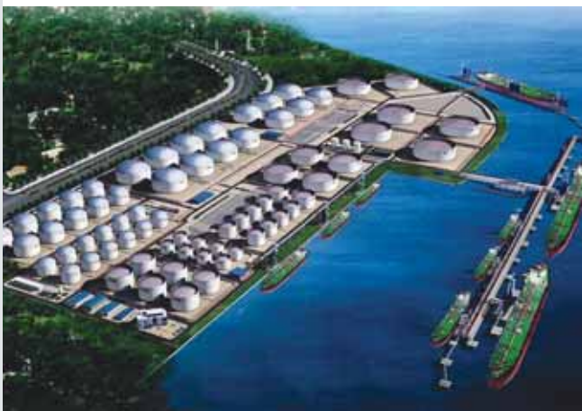
OKP completed its first and largest oil and gas-related project on Jurong Island.
