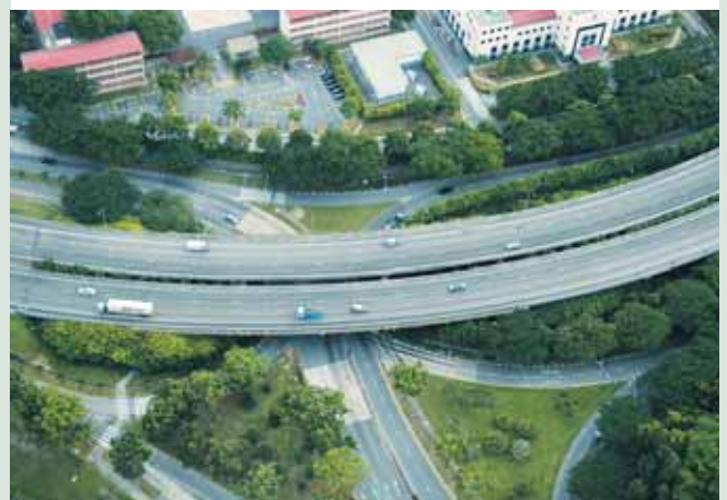
OKP's first design and build project at Bukit Timah Expressway.
