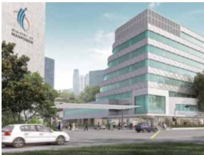
OKP constructed a covered linkway from the Ministry of Manpower building to Havelock Road in the Walk2Ride programme (ER443).
