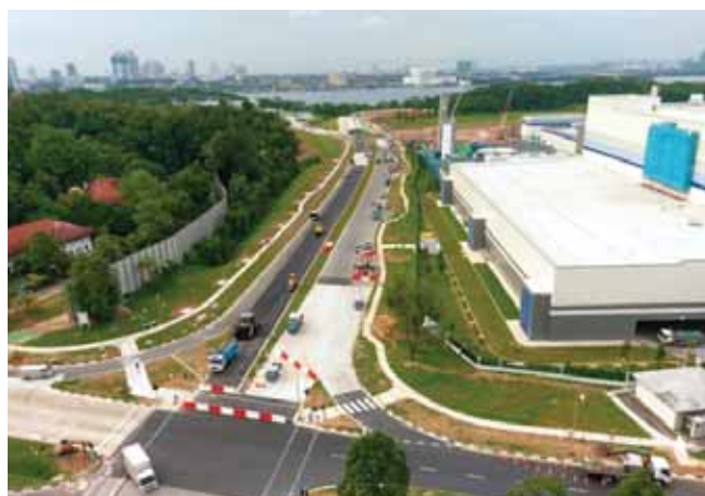
One of OKP's completed projects involved the extension of roads, drains and sewers works at Woodlands Avenue 4.
