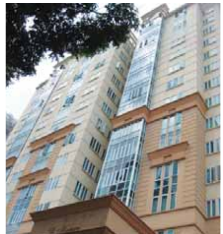
Another investment property, The Huntington at Moulmein Road.
