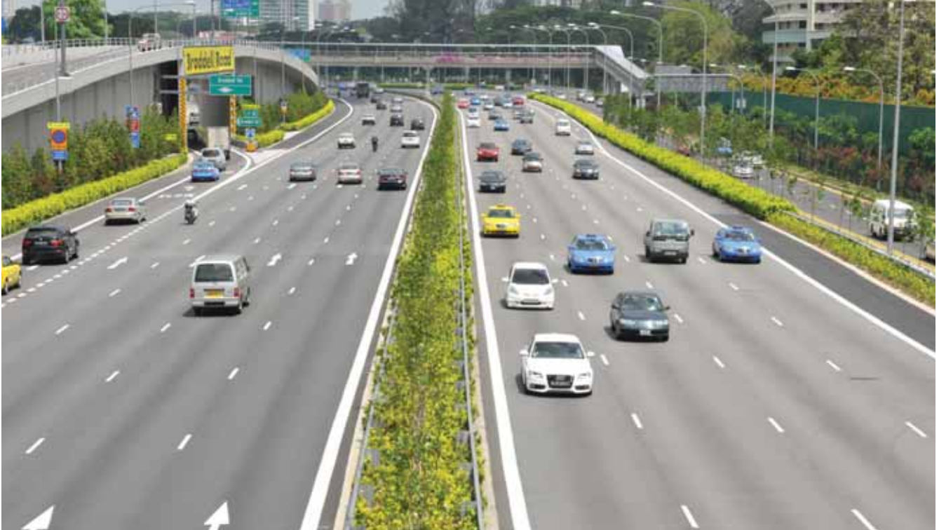
OKP completed the expansion of the CTE/TPE/SLE Interchange in 2015, one of the largest expressway projects in Singapore.
