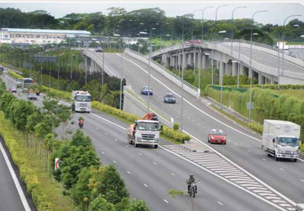
OKP designed and built the interchange at TPE/ Sengkang West Road/Seletar Aerospace Way.
