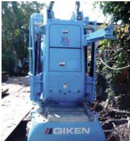
Newly purchased silent piler being used at our worksite.
