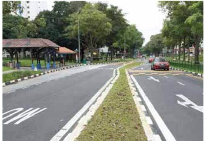
One of OKP's projects is the maintenance of road-related facilities, road structures and safety schemes in East Sector (Hougang Avenue 5 Silver Zone 4).
