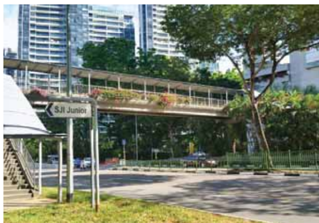
OKP completed a pedestrian overhead bridge at Novena in the Walk2Ride programme (ER443).
