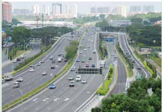
OKP's largest public sector project to date involved the widening of the CTE from PIE to Braddell Interchange.
