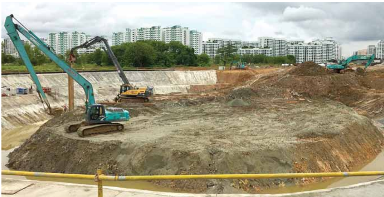
OKP started infrastructure works at Punggol (Phase 1) in 2016.
