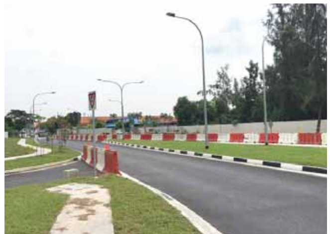
OKP is involved in the widening of Tanah Merah Coast Road.
