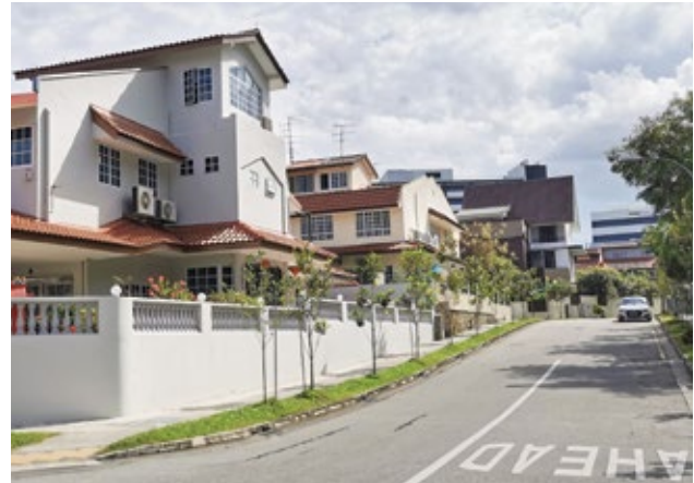
OKP has completed the maintenance of Pasir Ris Heights under the improvement to roadside drains V Contract E5.
