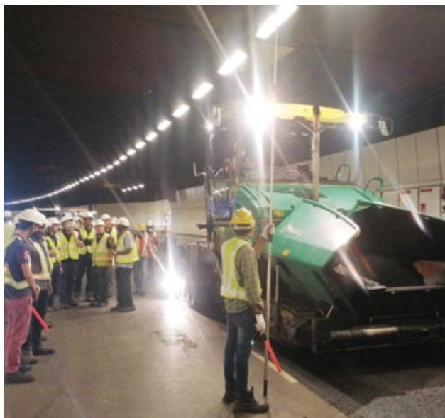
Site visit by customers at a road maintenance project for Expressway.
