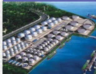
OKP completed its first and largest oil and gas-related project on Jurong Island.
