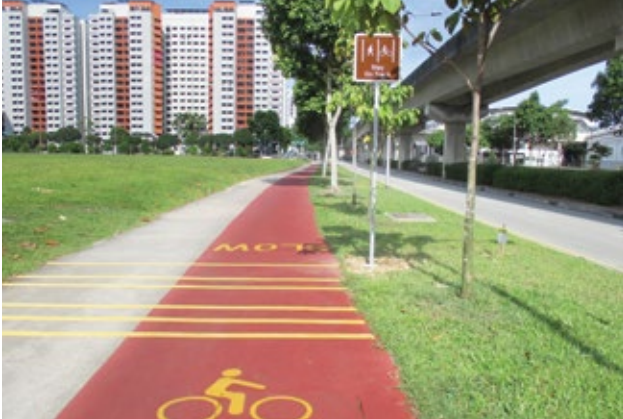
Cycling path at Sengkang East Avenue is one of OKP's ongoing maintenance projects under the term contract for road related facilities, road structures and road safety schemes for East Sector.
