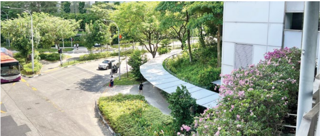
Under the Walk2Ride programme, OKP has completed the covered linkway at Jurong Gateway.
