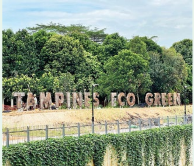
OKP completed the construction of Tampines Eco Green, part of Sungei Tampines project.
