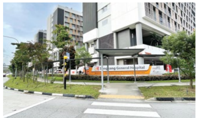
Under the Walk2Ride programme, OKP has completed the covered linkway at Sengkang East Way.
