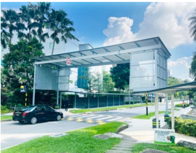
Under the Walk2Ride programme, OKP has completed the covered linkway at Anthony Road.
