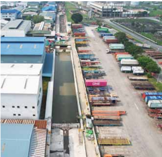
One of OKP's ongoing construction projects is the improvement to Benoi Road outlet drains.
