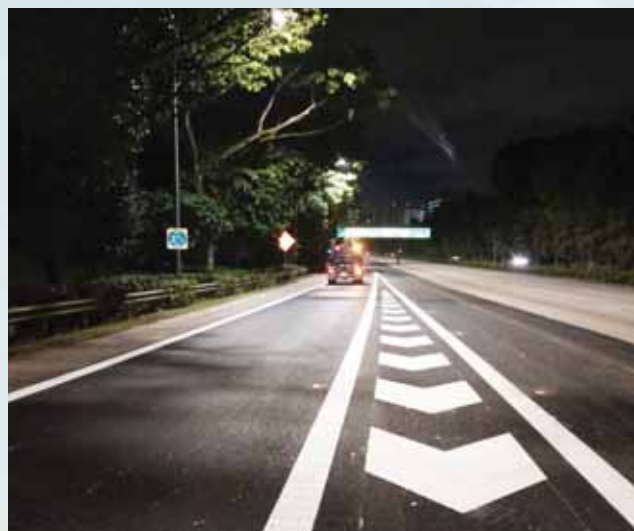
The Group completed the road maintenance contract for expressway.
