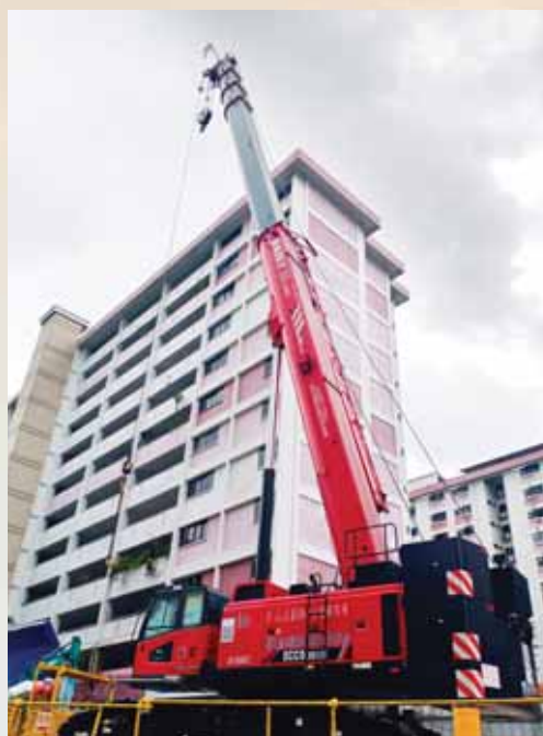
A newly purchased 90-ton telescopic crawler crane.
