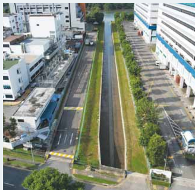
OKP has completed the improvement of West Coast outlet drain No. 6 (after Pandan Loop to the sea).
