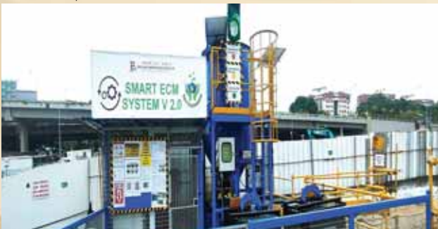
Our smart earth control measures system implemented at DEI43 project site.
