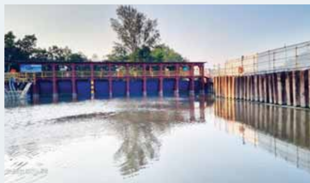
OKP is undertaking the improvement to Sungei Selarang and Sungei Selarang subsidiary drain A project.
