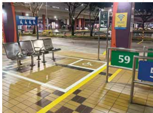
Commuter Infrastructure enhancement at Bishan is an ongoing OKP's construction project.
