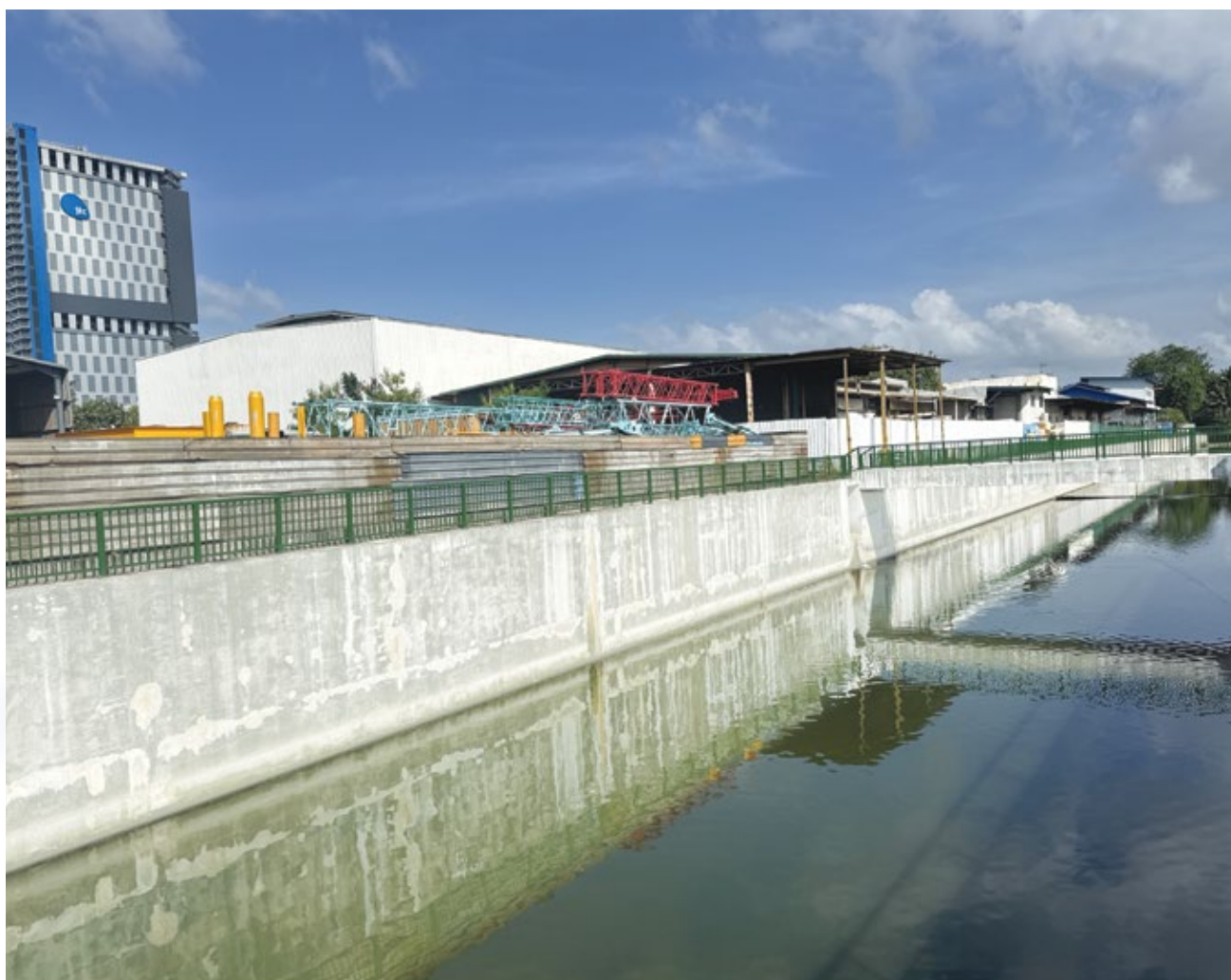
Improvement to Benoi Road outlet drains has been completed.
