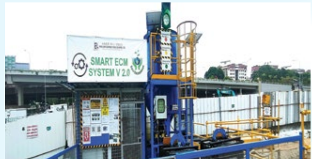
Our smart earth control measures system implemented at DE143 project site.
