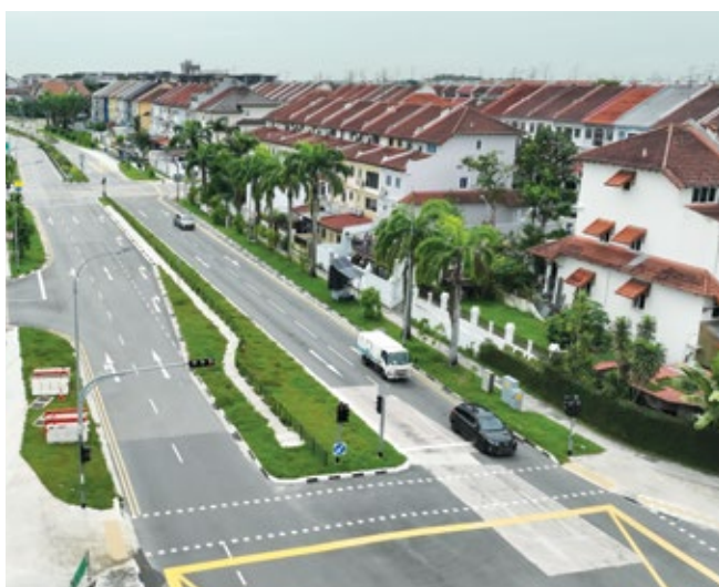
OKP is involved in the construction of commuter and road infrastructure works in Pasir Ris and Loyang.
