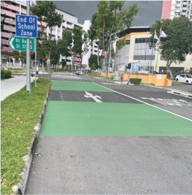
One of OKP's ongoing maintenance projects is the term contract for road-related facilities, road structures and road safety schemes for West Sector at Bukit Batok St 31's Friendly Street, which is designated for more convenient walking.
