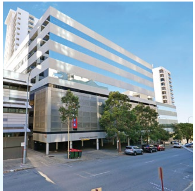
Exterior view of 6-8 Bennett Street in East Perth, Western Australia.
