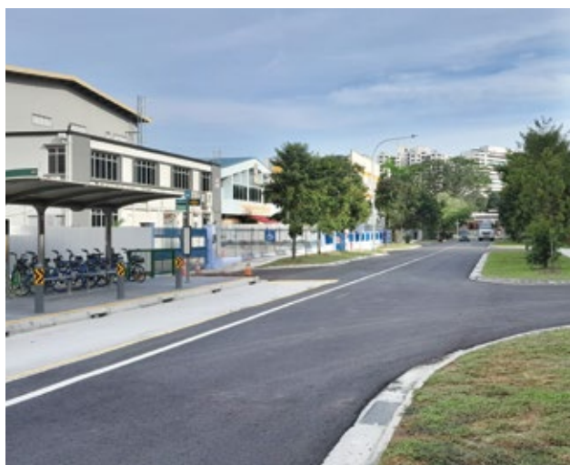
Improvement to roadside drains at Jalan Teliti, Toh Tuck Road, Jalan Senang, Pasir Panjang Hill and Enterprise Road is an ongoing OKP's maintenance project.
