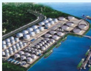
OKP completed its first and largest oil and gas-related project on Jurong Island.
