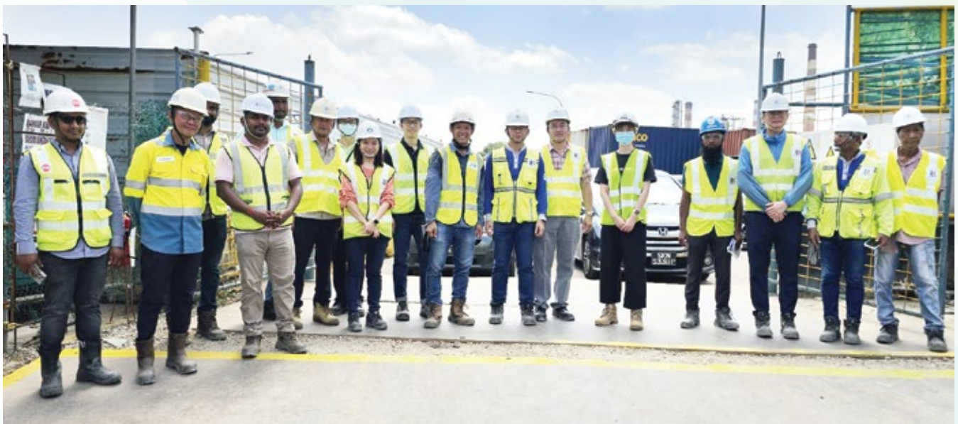
Our teams conducting a cross audit together with PUB at an OKP's construction site on 25 March 2024.
