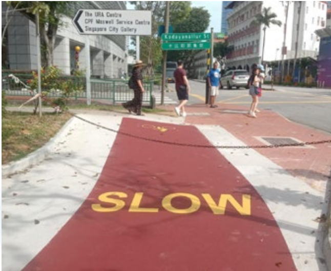
Completed work using carbon mineralised concrete for the construction of the Cycling Path Network at Maxwell Road.
