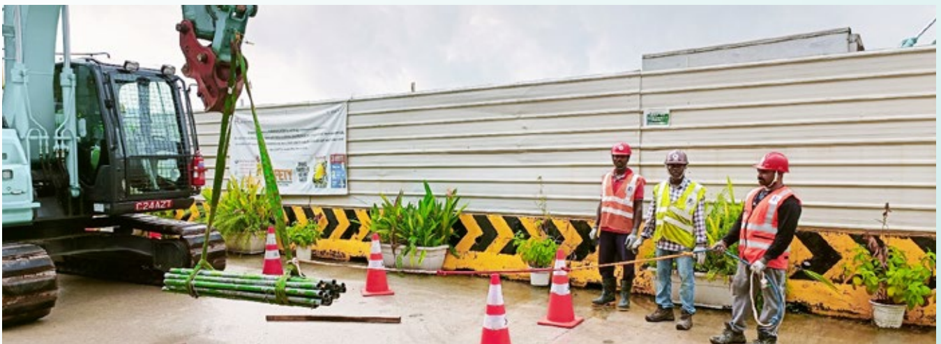
Briefing on safe lifting on-site.
