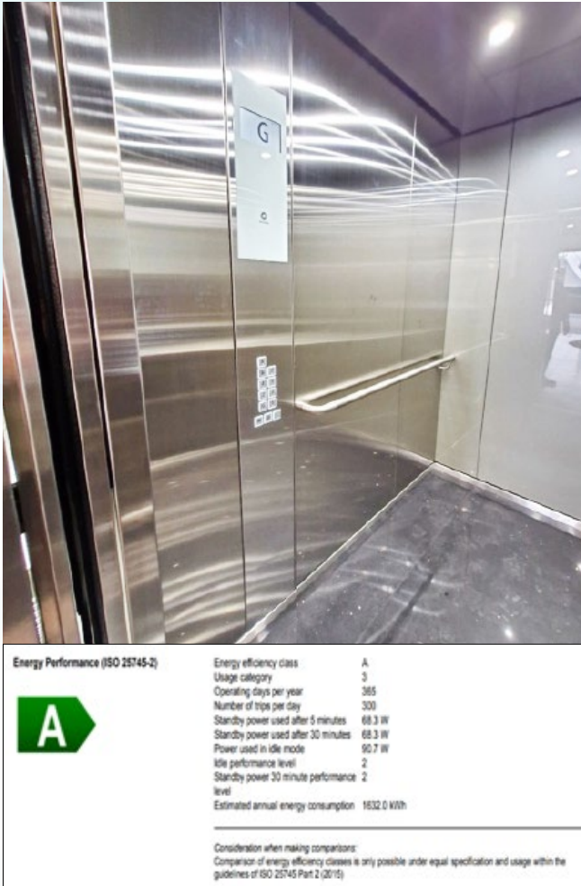
New energy performance rated A lifts installed at Perth office complex.
